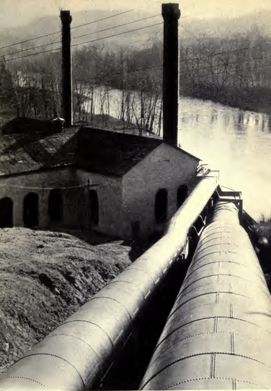
HYDROELECTRIC PLANT, BULLS BRIDGE
